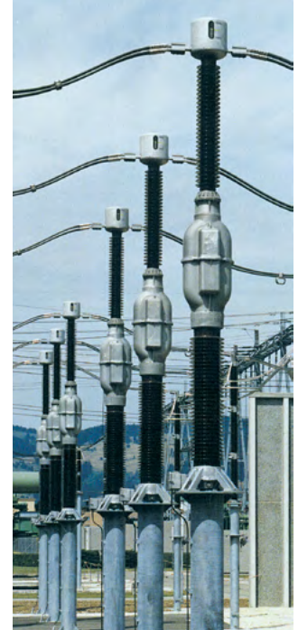
Fig. 4.2-17: 420 kV oil-paper-insulated inductive voltage transformers
