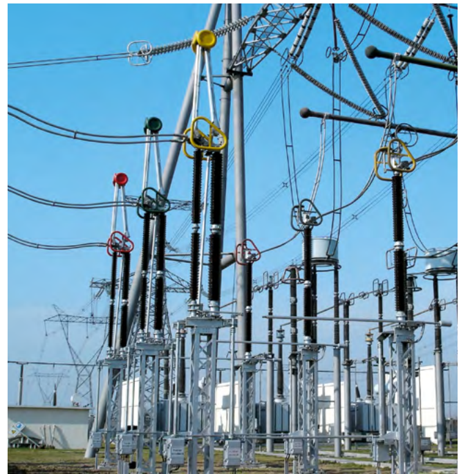
Fig. 4.1-29: Knee-type disconnector
