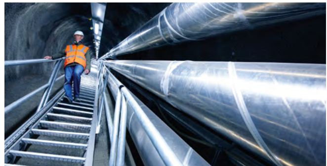
Fig. 2.2-49: GIL laid in shaft with 42° gradient (Limberg, Kaprun, Austria)
