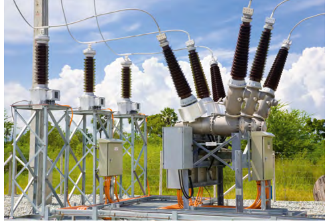
Fig 3.1-27: Dead Tank Compact (DTC)
