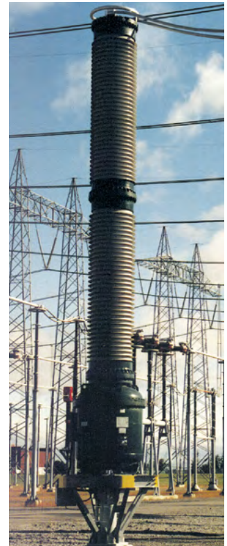
Fig. 4.2-14: 800 kV gas-insulated current transformers
