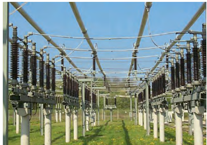
Fig. 3.1-14: Busbar disconnectors "in line", 110 kV, Germany
