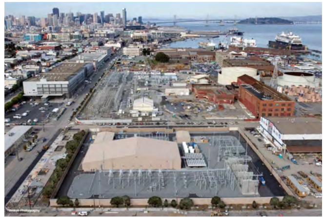
Fig. 2.2-6: Converter station of the TransBay Project close to the city center of San Francisco. The world's first VSC HVDC transmission scheme in modular multi-level converter (MMC) topology
