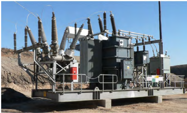
Fig. 2.4-14: 145kV 10MVA skid substation
