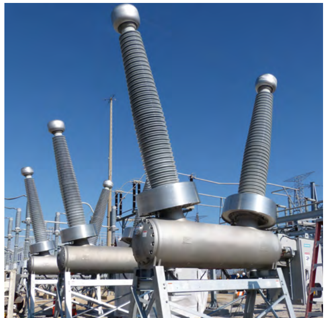
Fig. 4.1-13: SPS2/3AP1 DT 362 kV (two cycles)
