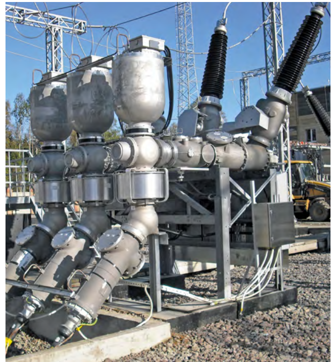
Fig. 4.1-20: 3AP1 DTC 145 kV with voltage transformer and cable connection
