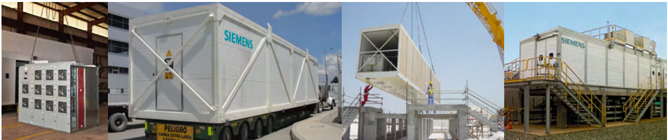
Fig. 2.4-4: E-House: Completely developed, manufactured, assembled and pre-tested at factory, shipped as one single unit or in splitting sections, installed, connected and commissioned on site
