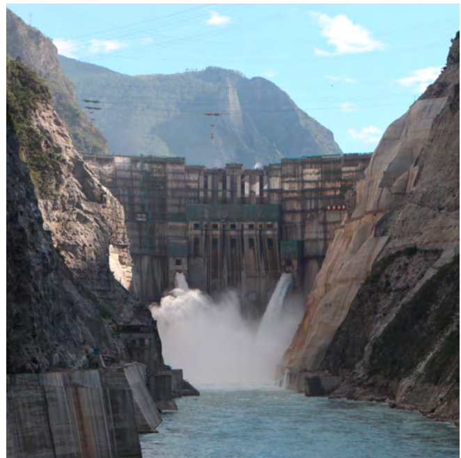
Fig. 2.2-52: Jinping, China, the world's tallest HPP dam
