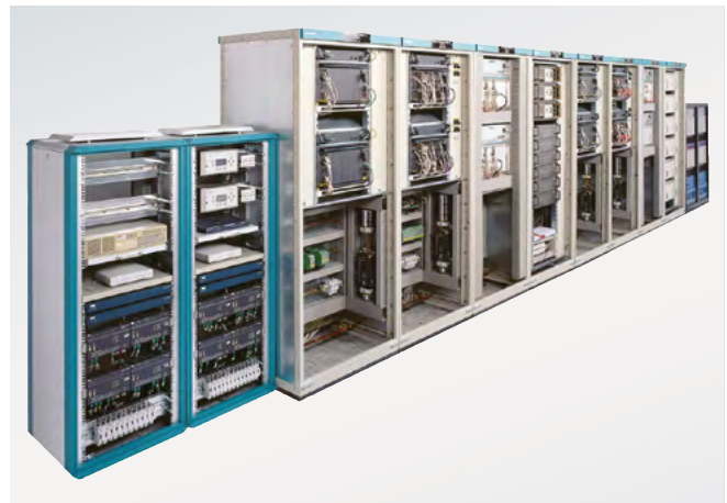
Fig. 2.2-17: The control and protection cubicles are intensively tested in the Siemens laboratories before they are shipped to site, assuring fast and smooth commissioning of the HVDC system
