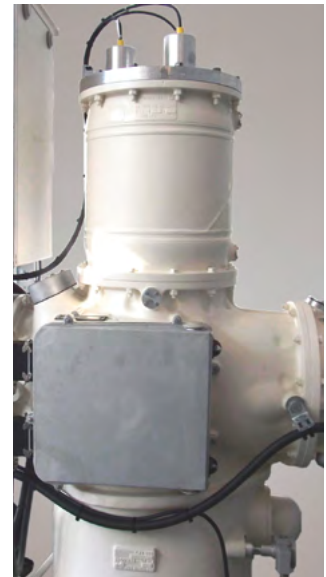
Fig. 4.2-24: 145 kV RC divider for GIS
