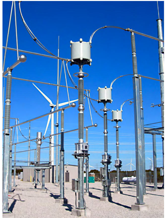
Fig. 4.2-33: Line traps
