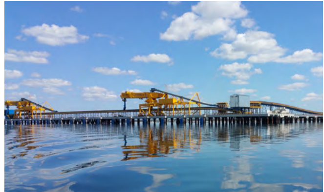
Fig. 2.4-9: E-house for the Nacala-a-Velha port in Mozambique
