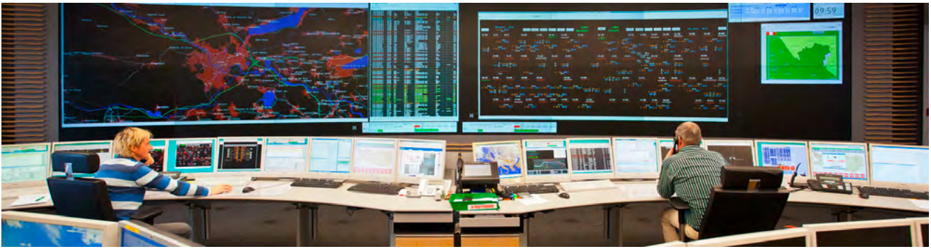
Fig. 7.1-24: Typical control room environment
