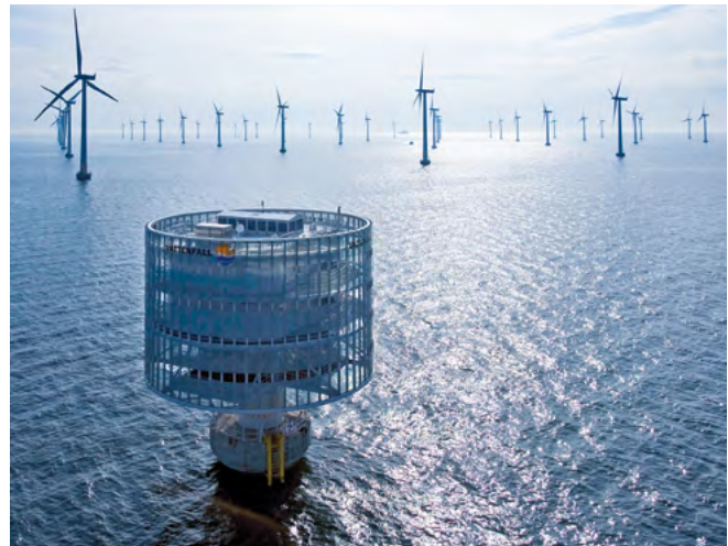
Fig. 2.2-30: 2007 110 MW Offshore Wind Farm Lillgrund, Sweden
