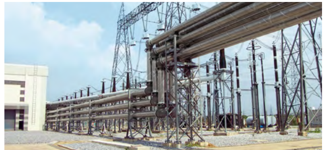
Fig. 2.2-45: Above ground installation
