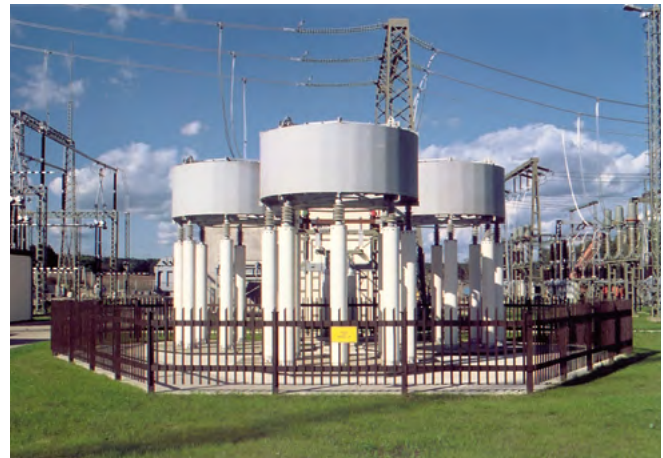
Fig. 4.2-35: Tertiary-connected shunt reactors
