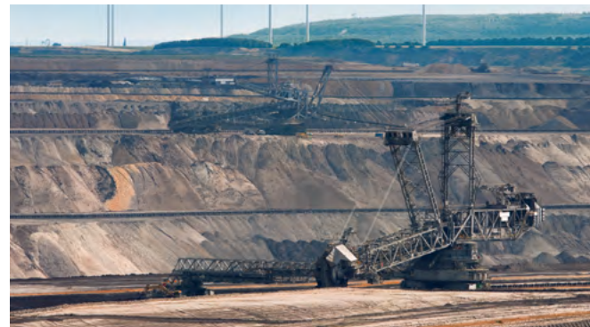
Fig. 2.5-5: Critical infrastructures microgrids – renewable energies in critical environments
