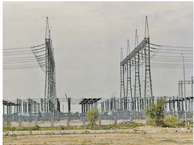
Fig. 3.1-20: One-breaker-and-a-half arrangement, 500 kV, Pakistan
