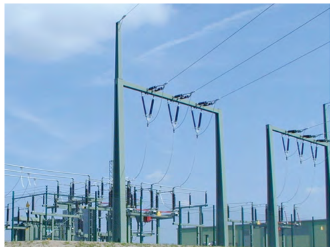
Fig. 3.1-12: H-arrangement, 110 kV, Germany
