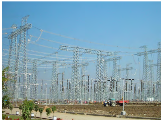
Fig. 3.1-22: One-breaker-and-a-half arrangement, 800 kV, India
