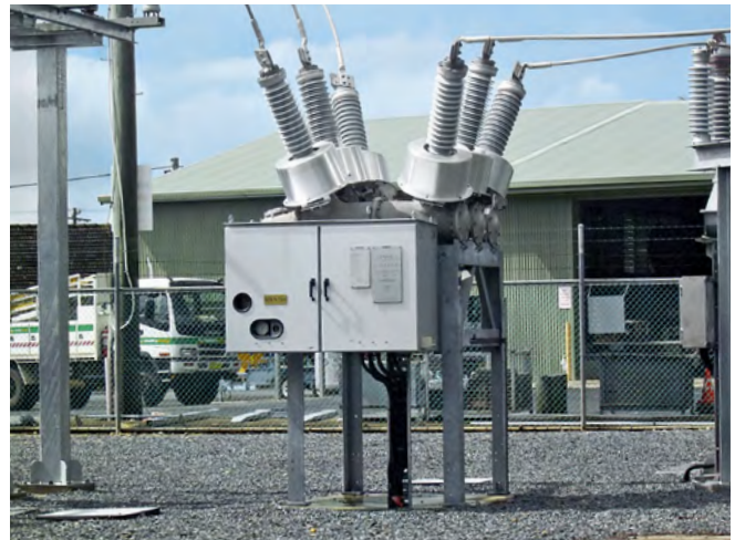
Fig. 4.1-11: SPS2/3AP1 DT 72.5 kV
