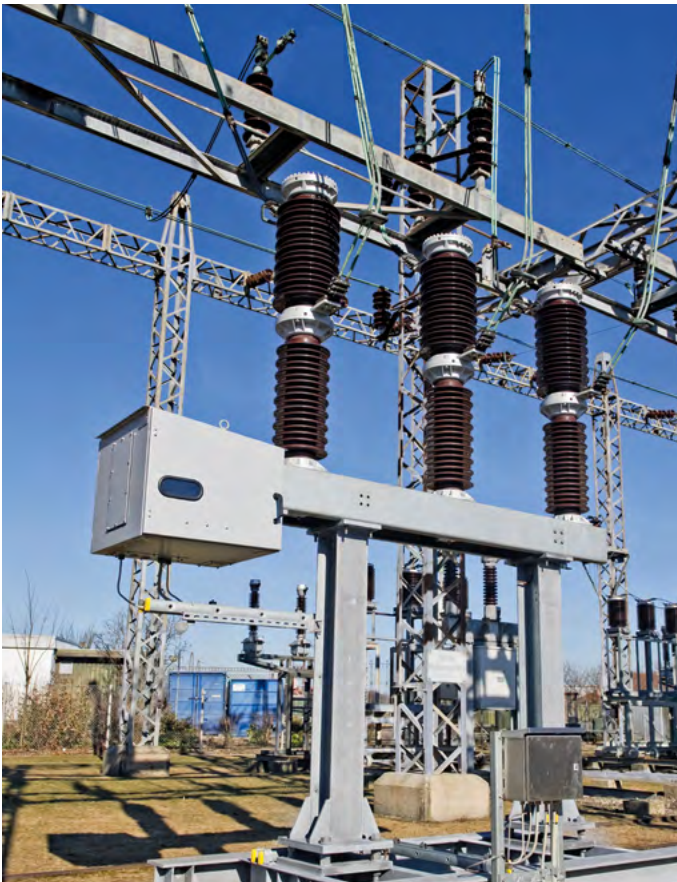
Fig. 4.1-10: 3AV1 FG vacuum circuit-breaker 72.5 kV
