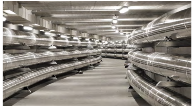
Fig. 2.2-46: GIL tunnel installation, Munich, Germany
