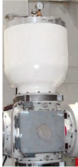
Fig. 4.2-27: 145 kV inductive voltage transformer for GIS
