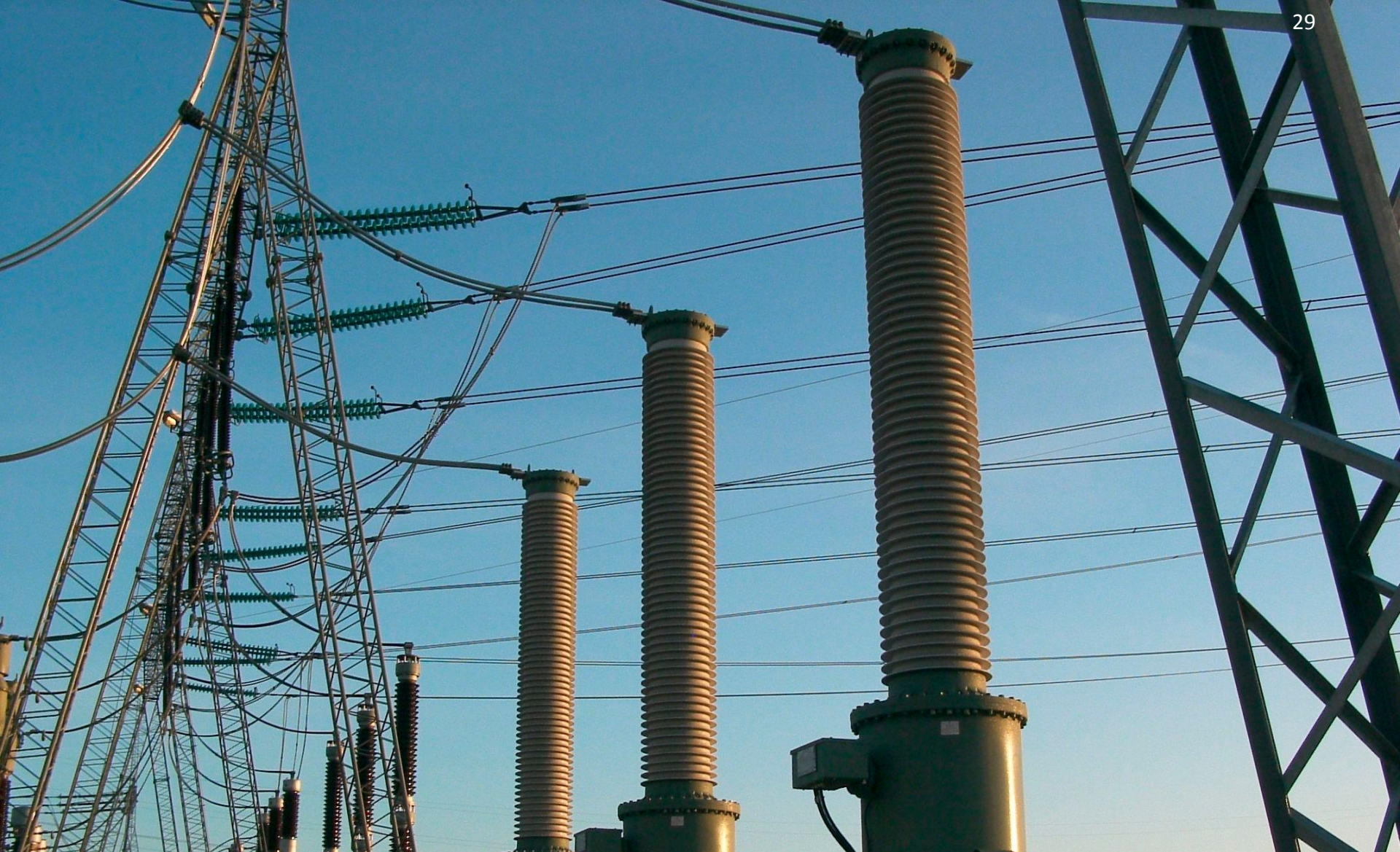
Voltage Measuring Transformers (VT)
