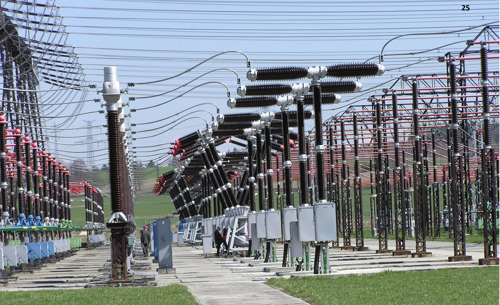
SF 6 Gas-filled Circuit Breaker
