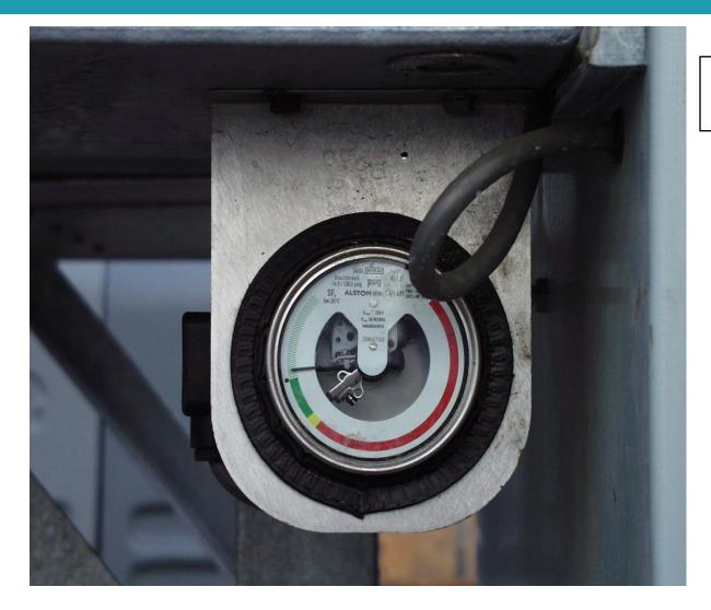
SF6 pressure gauge on 115kV CB (Alstom)
