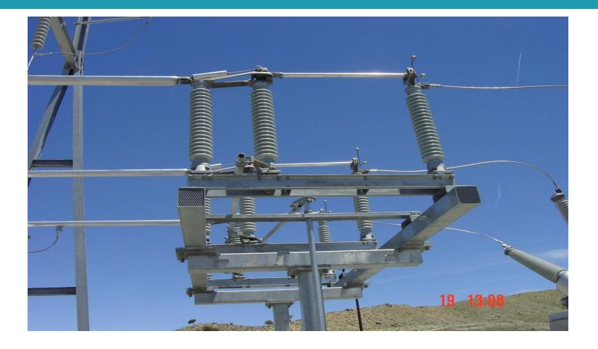
A special type of high-voltage disconnect switch is the ground switch. Ground switches are disconnect switches that provide a solid ground to a power line or piece of station equipment such as a bank or a bus. The general function of a ground switch is to provide a safety ground.
