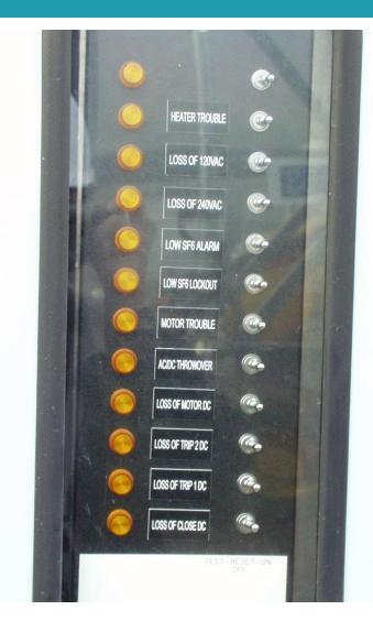
Annunciator Panel located on the breaker. 115kV CB (Alstom)
