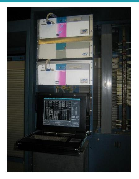
Digital Fault Recorder mounted in a 225kV station.
