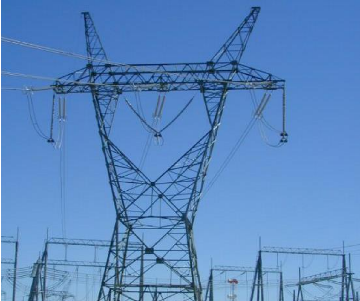
Steel Lattice 500kV Tower
