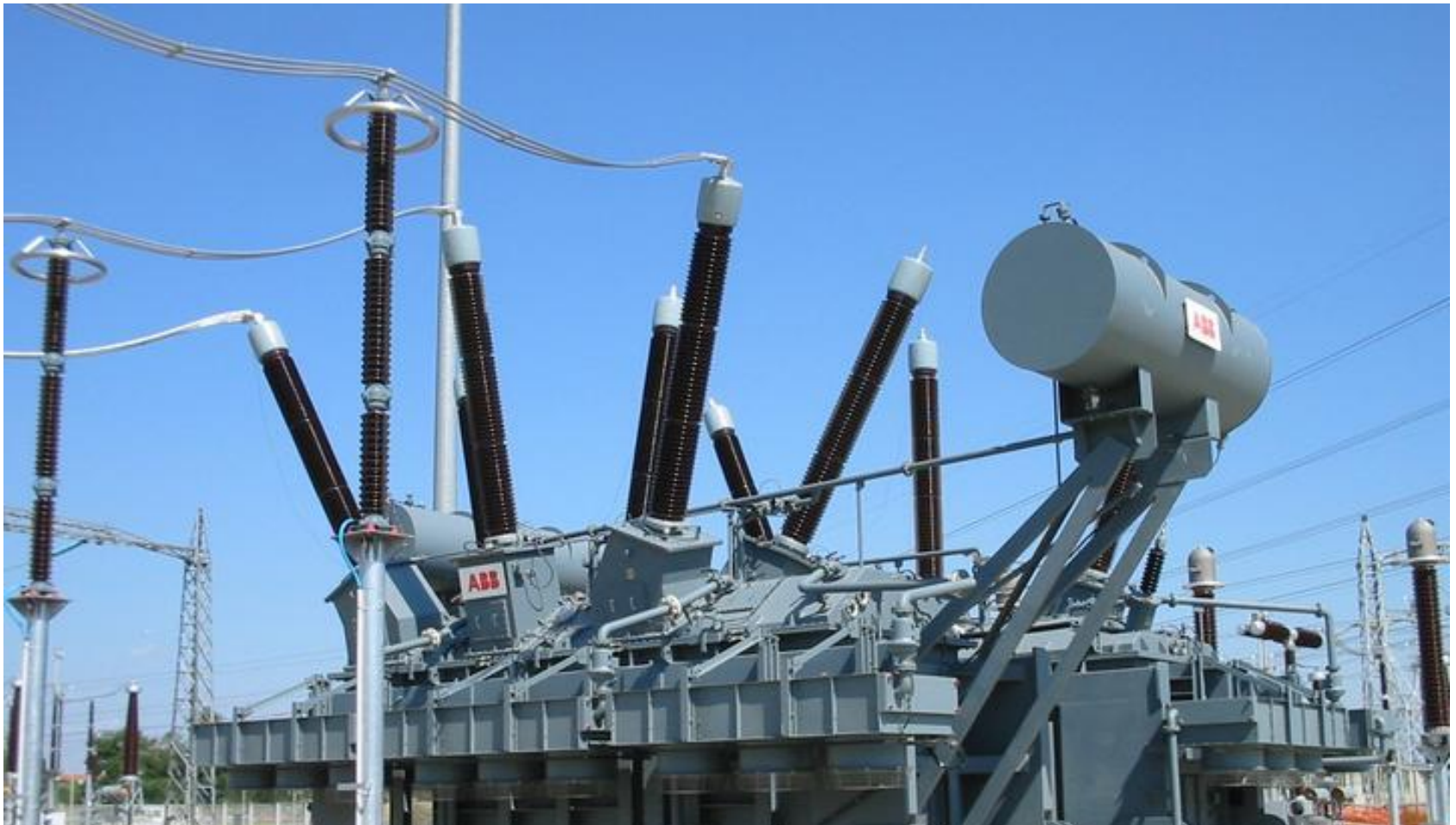
Phase Shifting Transformer – “Phase Shifter”
