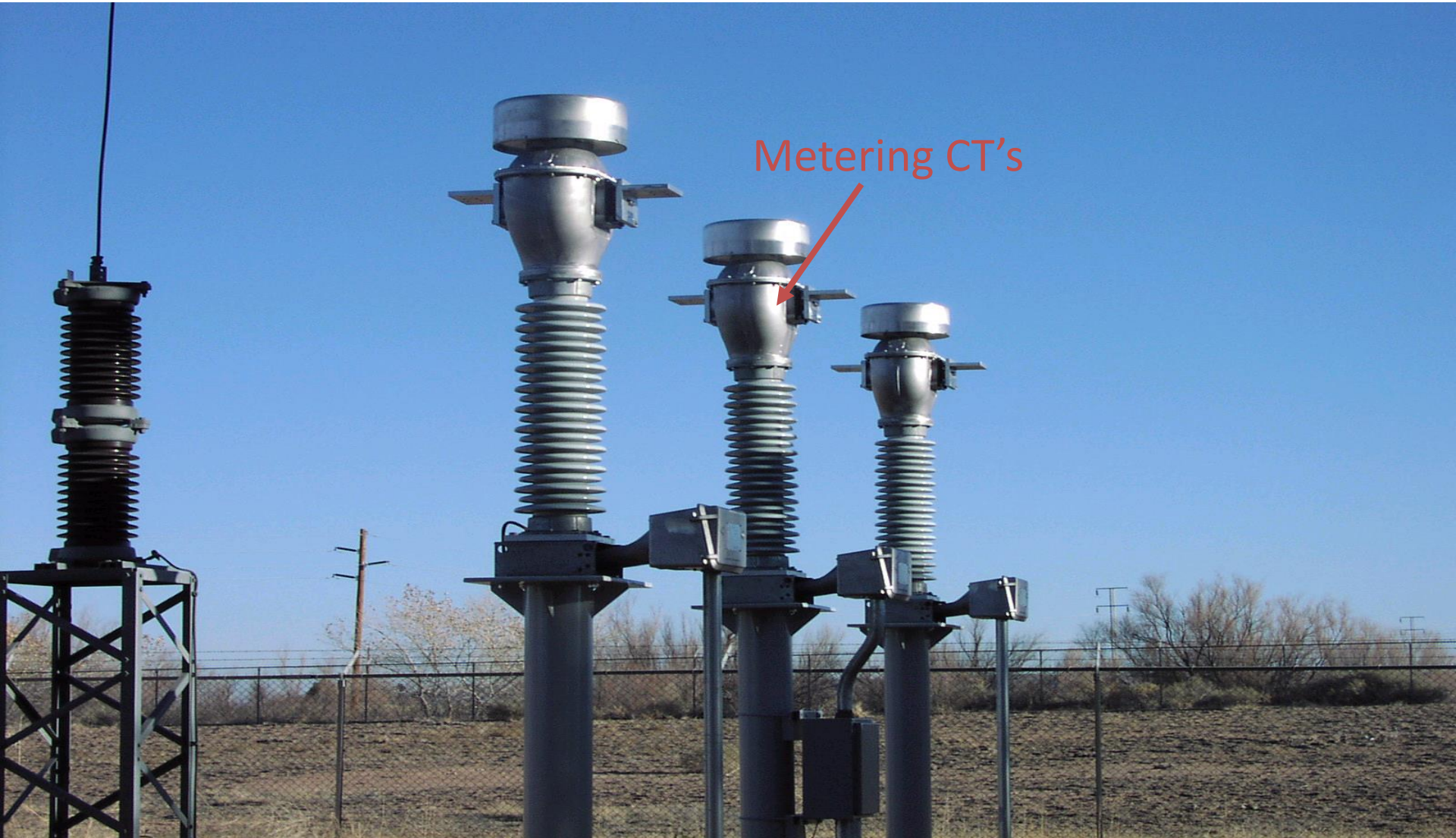
Current Transformer (External)
